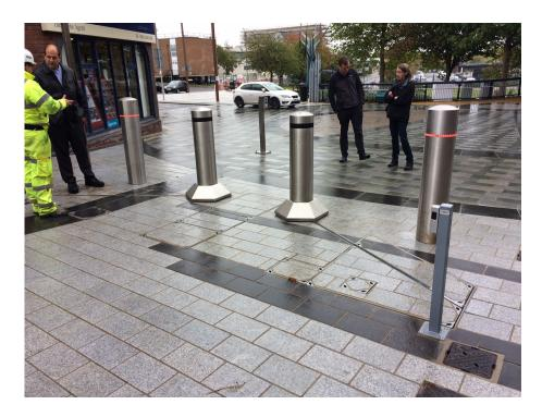
Bollards with inset paving finish to the surface.
